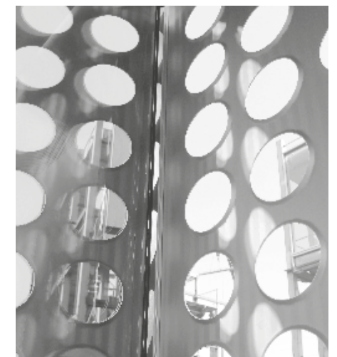
Screens punched with Prouvé-inspired portholes reduce solar load and protect from wind
