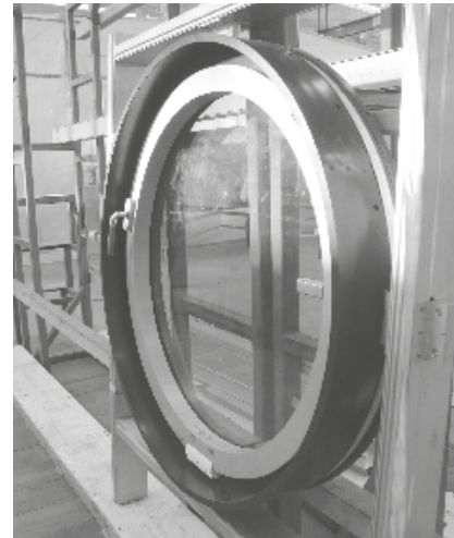
Porthole-shaped openable windows naturally ventilate office floors
