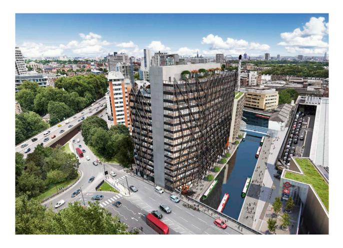
On completion in the first half of 2019, Brunel Building will total 243,000 sq ft with an exciting external diagrid structure creating generous 3.5m tall largely column-free 17,000 sq ft floorplates. The ground floor will have a spacious canalside reception as well as restaurant/café space, and in addition the building will benefit from two large rooftop terraces. The project will open up new public access to Paddington Basin and is sited opposite an entrance to the Elizabeth line.
