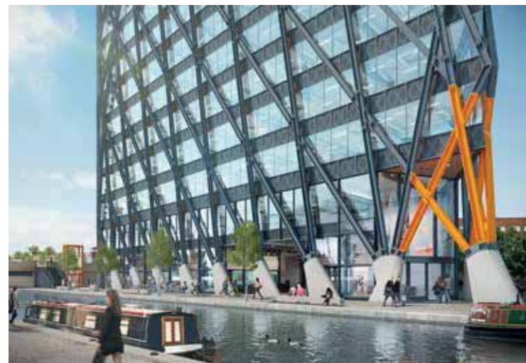
Brunel Building W2
