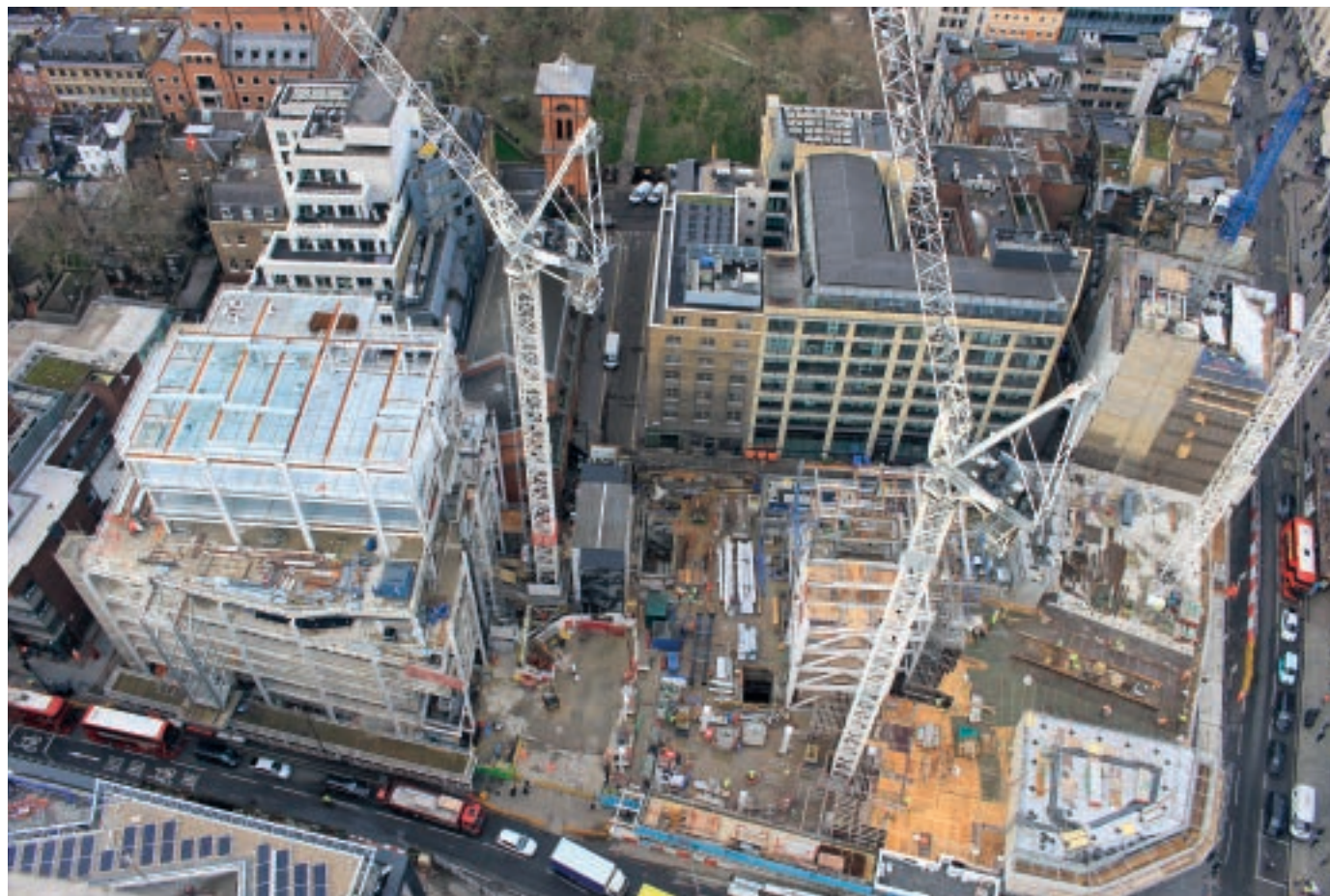
Soho Place site
