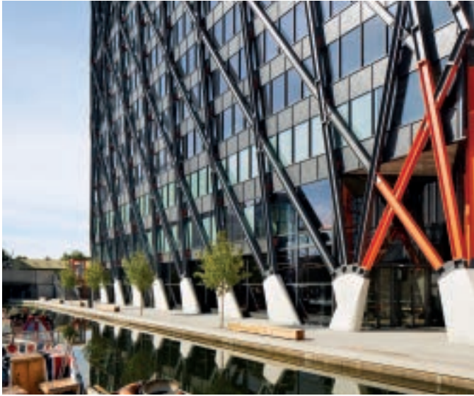
Brunel Building W2 – completed in May 2019
