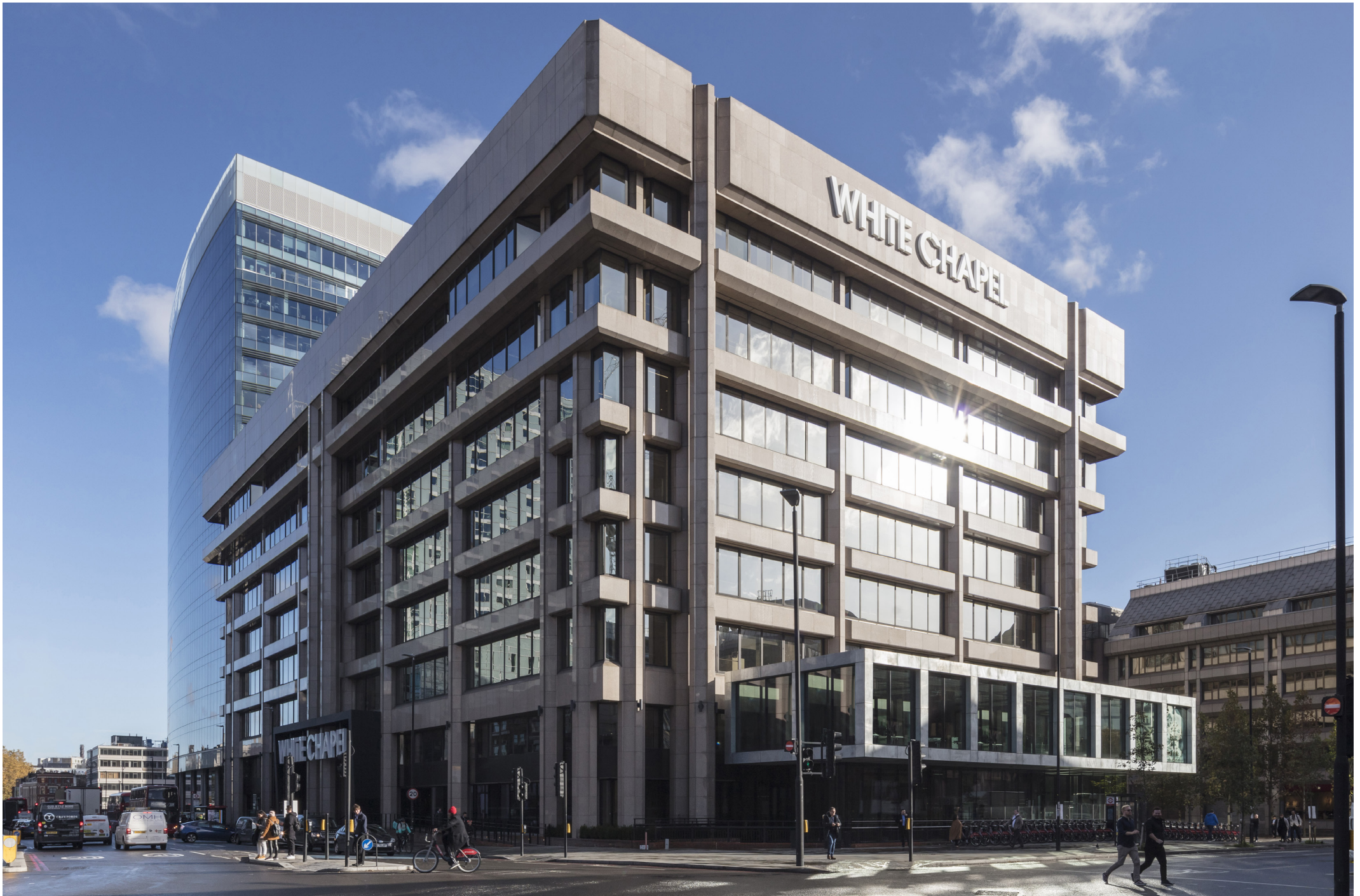
THE WHITE CHAPEL BUILDING
