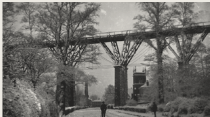
One of Brunel’s now lost timber viaducts spanning the Great Western Railway
