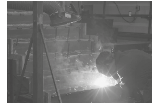
Chay Wheeler on site welding the suspended stair
