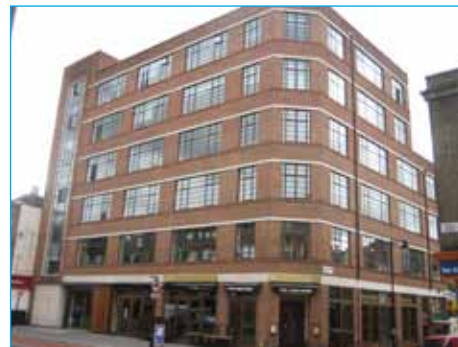
Suncourt House N1
