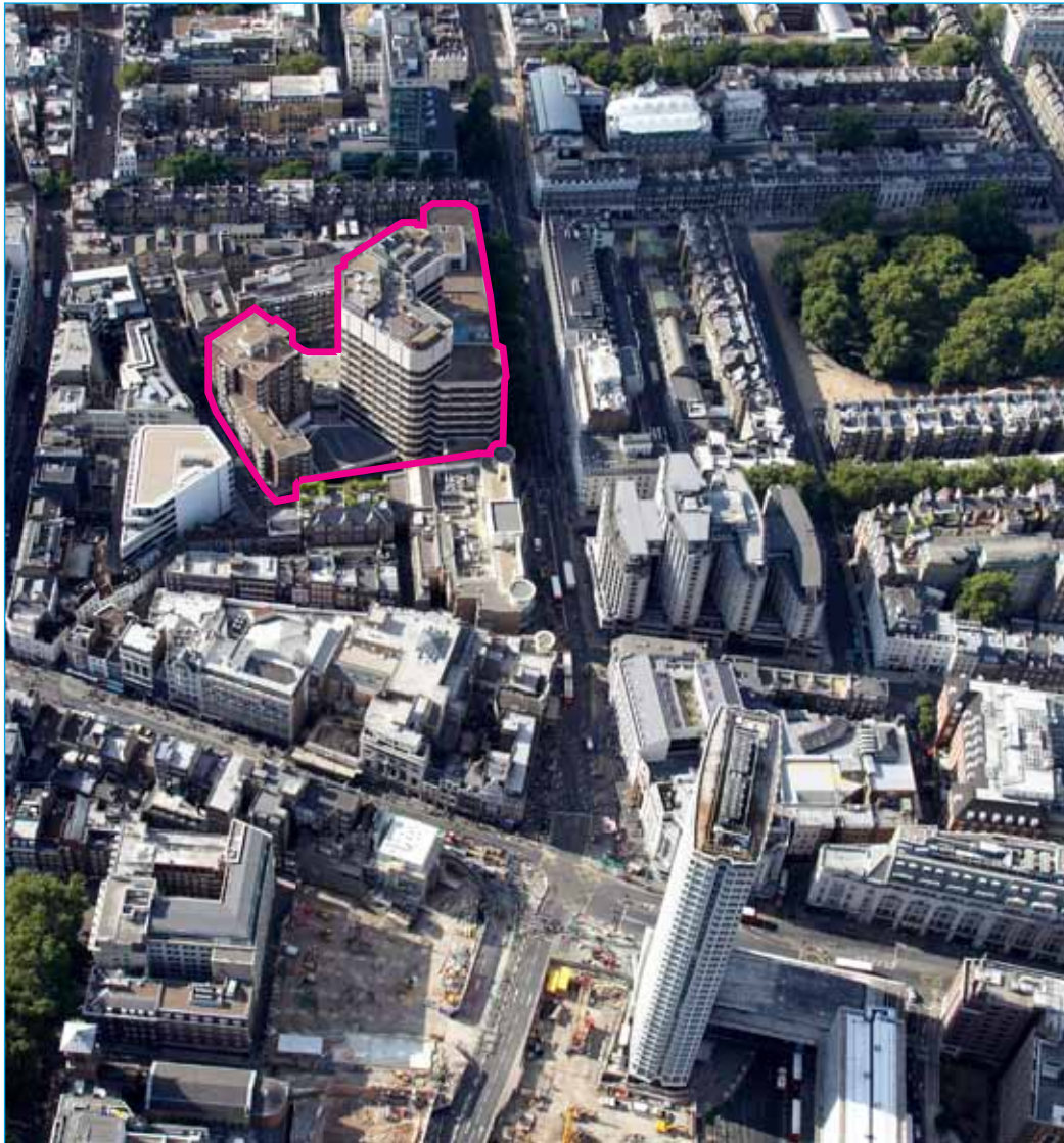
Central Cross, 18-30 Tottenham Court Road W1
