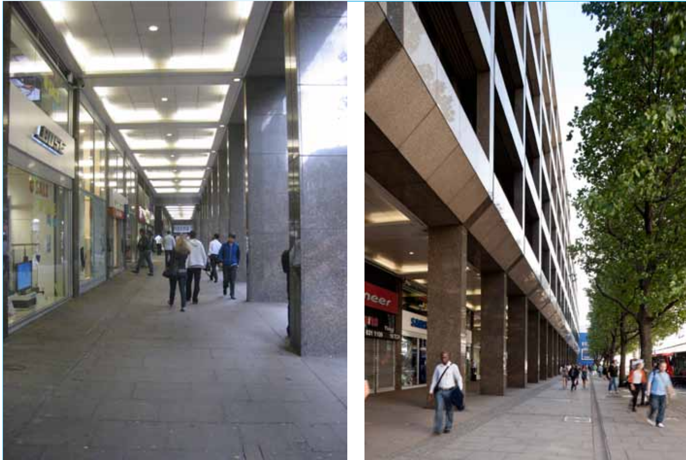
Existing retail frontage: Tottenham Court Road
