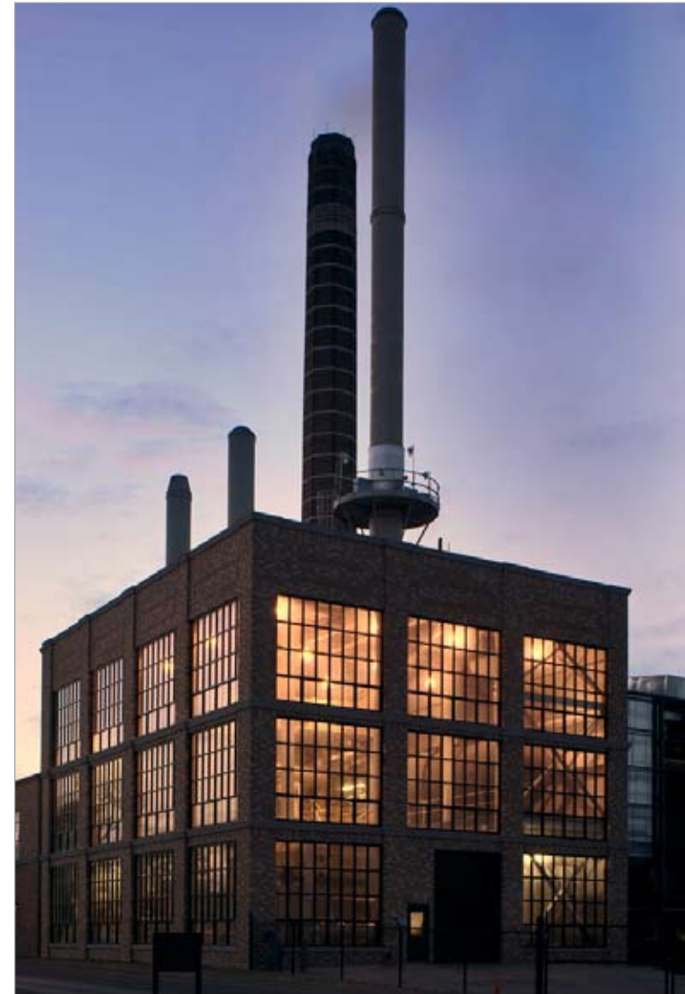
Boiler House, University of Notre Dame (1985)
